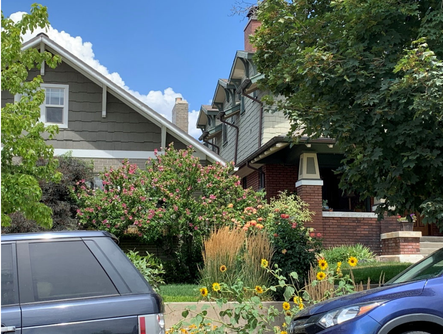
The two-story home on the right is an example of a vertical inline addition special exception. The existing home did not meet current side yard setbacks.
