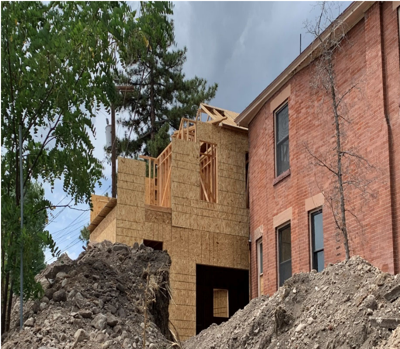
The Historic Landmark Commission approved additional height for the addition on this historic home in the Avenues.
