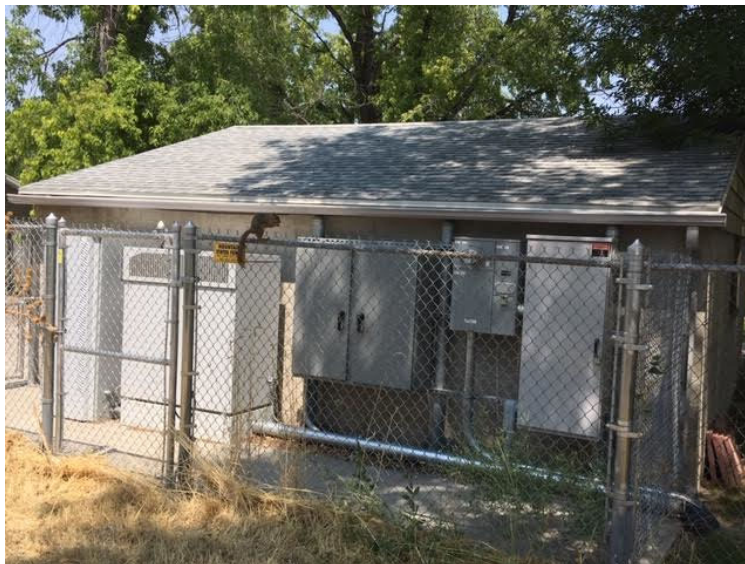
Cell tower electrical equipment on an accessory building next to the 9Line. This change would require this equipment to be screened with a solid fence or wall.
